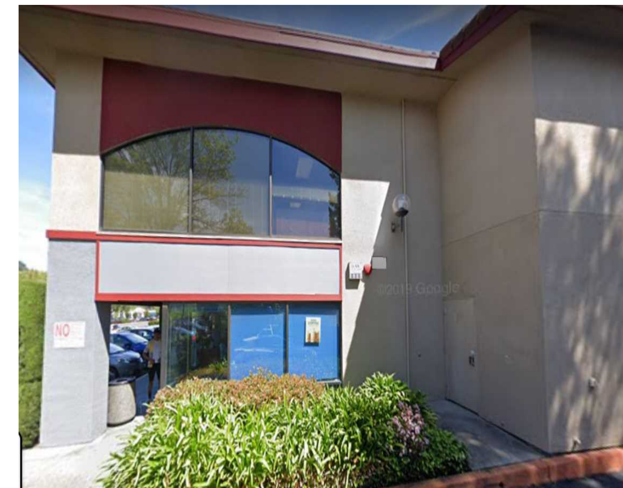
G SIDE OF EXISTING OFFICE BUILDING
